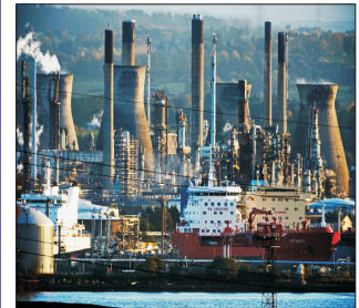
Refinery Petrochemical Plant
